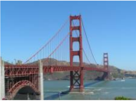
Golden Gate Bridge
